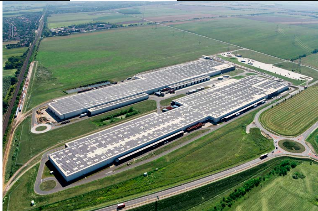
Audi Hungaria: photovoltaic system on the roofs of the two logistics halls.
